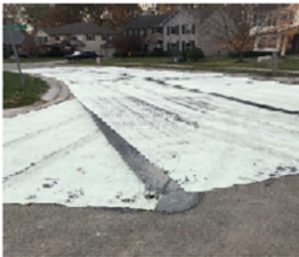
Figure 1: Burberry Place – Road Fabric placement
