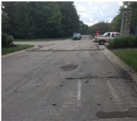
Figure 1: Curb Ramp Work in Hawthorne Ridge
