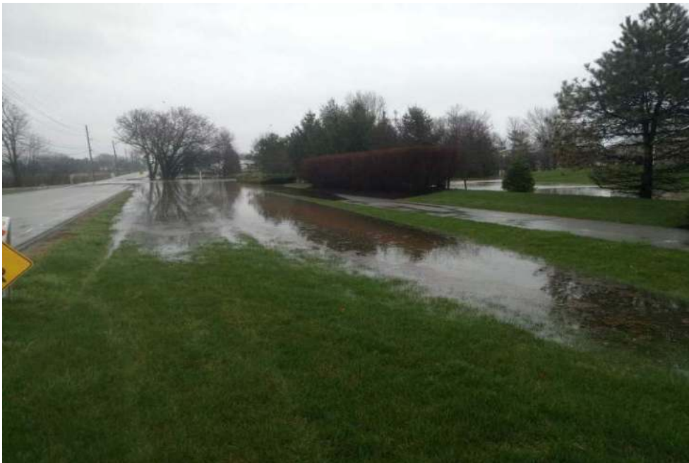
Photograph No. 32 Looking East along the South side of 136th St
