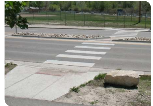
Curb ramps must include truncated domes. Sedimentation and snow accumulation are challenges.
