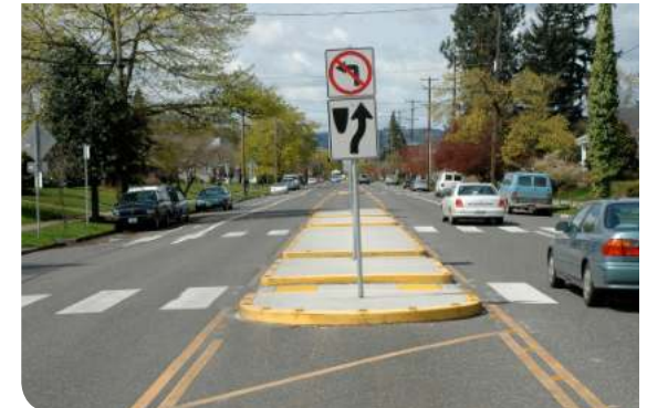
This crossing island doubles as a partial diverter. Curb ramps are “cut through,” allowing pedestrians to remain at-grade.
