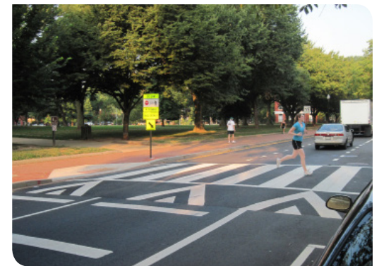
Raised crosswalks have traffic-calming effects. This crosswalk crosses two travel lanes, a bike lane, and a parking lane.
