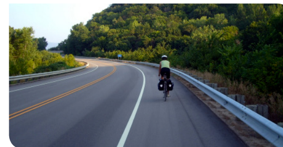
Wide paved shoulders reduce run-off-road crashes, improve roadway maintenance, and can provide space for bicyclists.
