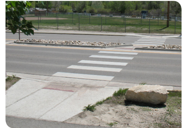
Curb ramps must include truncated domes. Sedimentation and snow accumulation are challenges.
