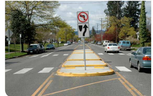
This crossing island doubles as a partial diverter. Curb ramps are “cut through,” allowing pedestrians to remain at-grade.
