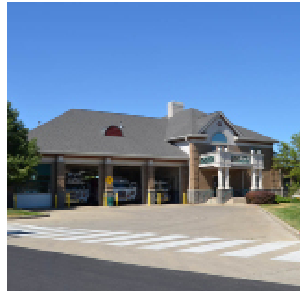
Municipal Center: Fire Station
