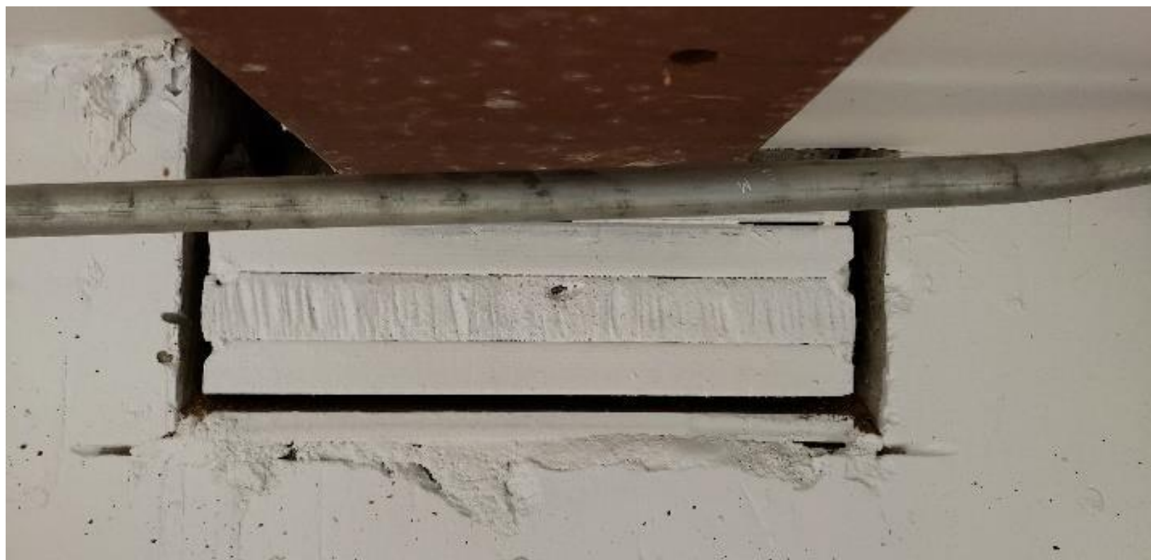
Steel wide-flange beam with gap between the bearing surface of the pocket
