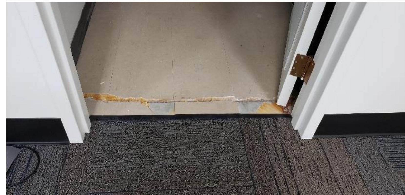
Cracked floor tiles at door threshold to the server room at the second floor
