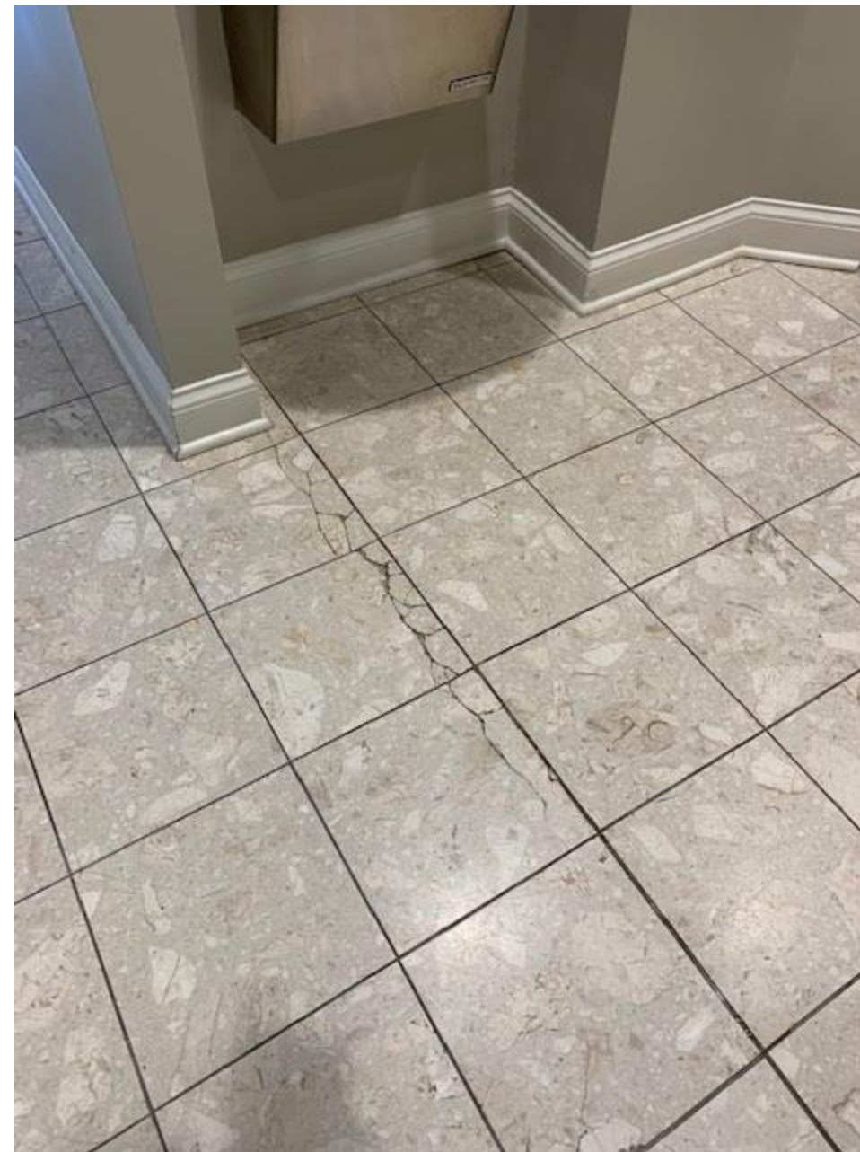
First Floor Interior West Side water fountain Flooring sagging significantly
