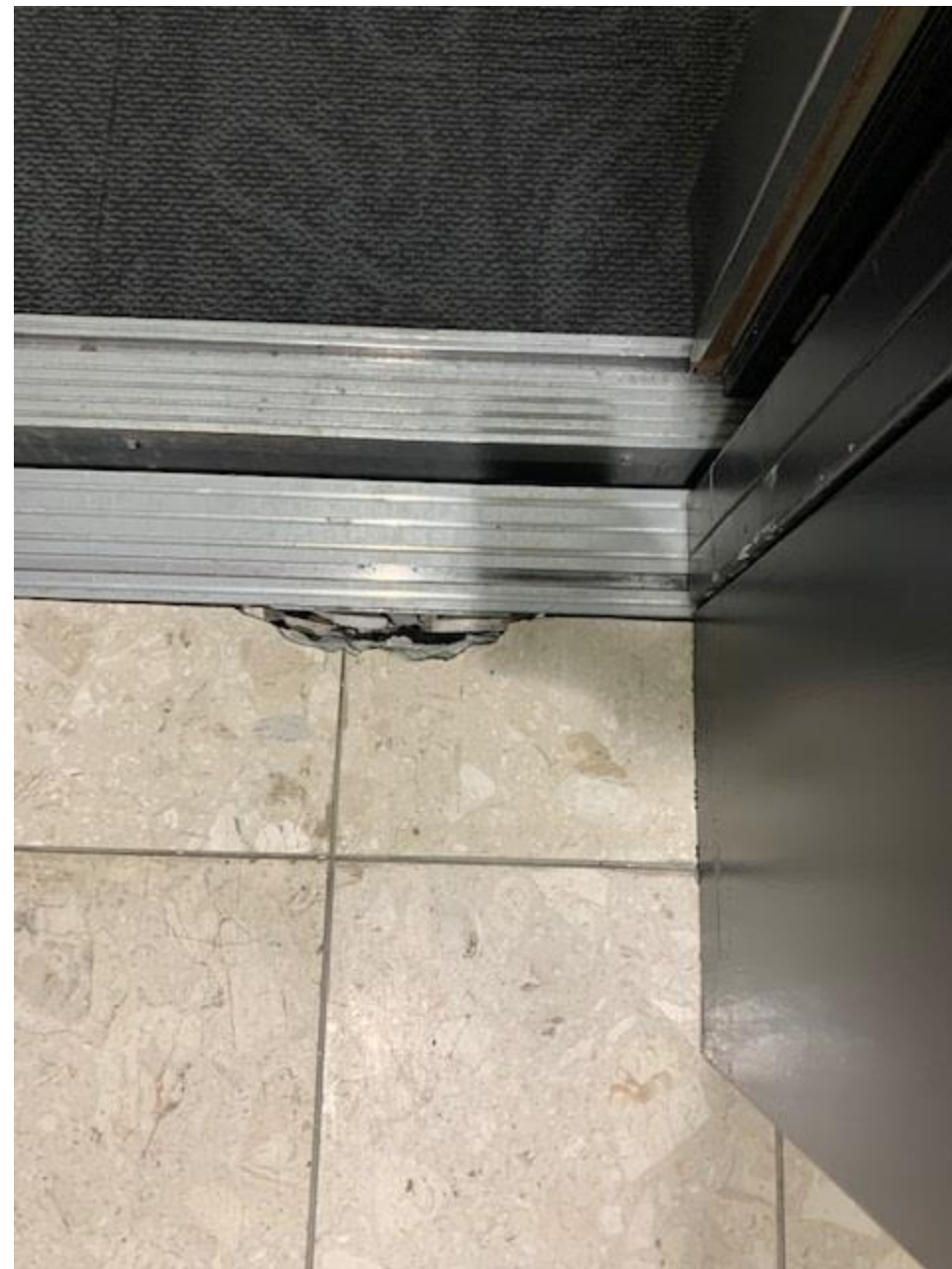
Second Floor Interior West Side Elevator Flooring breaking apart
