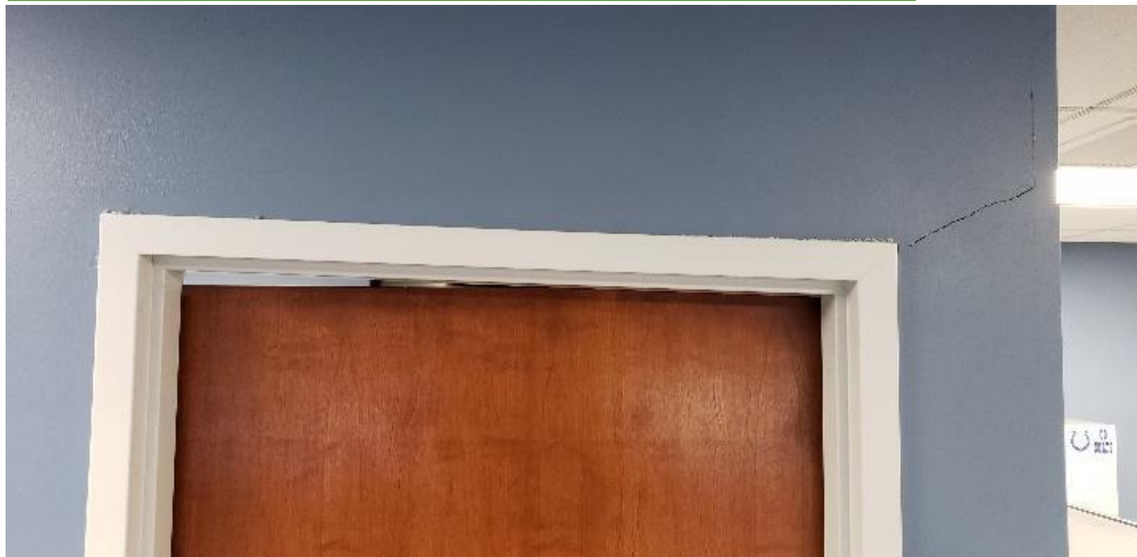
Crack in wall widened at increasing height
