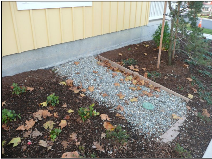
Figure 1 Infiltration Bed, Seattle, WA (USEPA, picasaweb)
