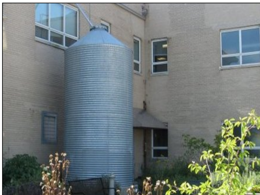
Figure 1 Above ground cistern, Chicago, IL (USEPA, picasaweb)
