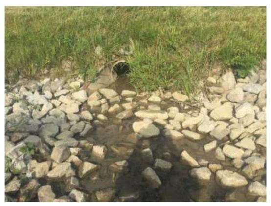
119. Looking west at 16-inch diameter culvert under SR 37 that likely drains into Wetland P.
