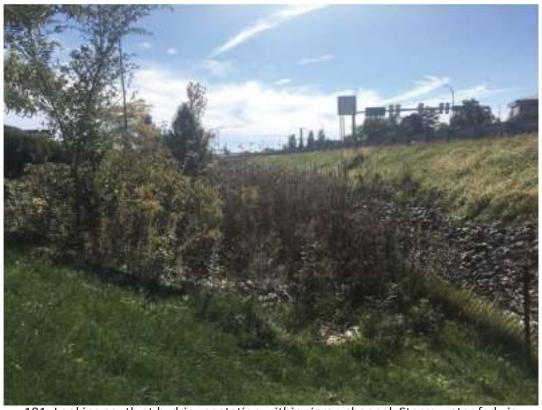
191. Looking south at hydric vegetation within riprap channel. Storm water fed via culvert drainage from parking lot.
