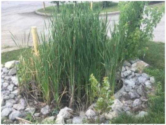
122. Looking north towards small storm water ponding area. No soil indicators exist as cattails are growing directly out of riprap.
