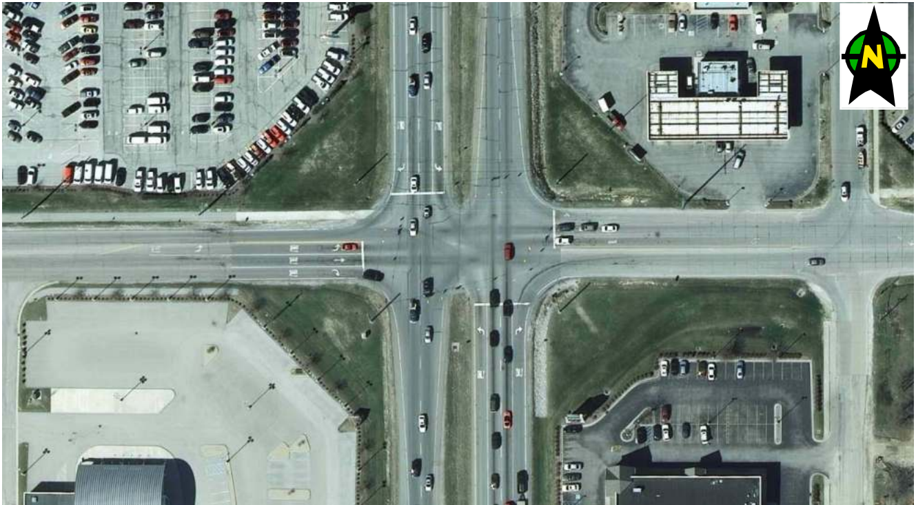
Intersection of SR 37 and 126 th Street
