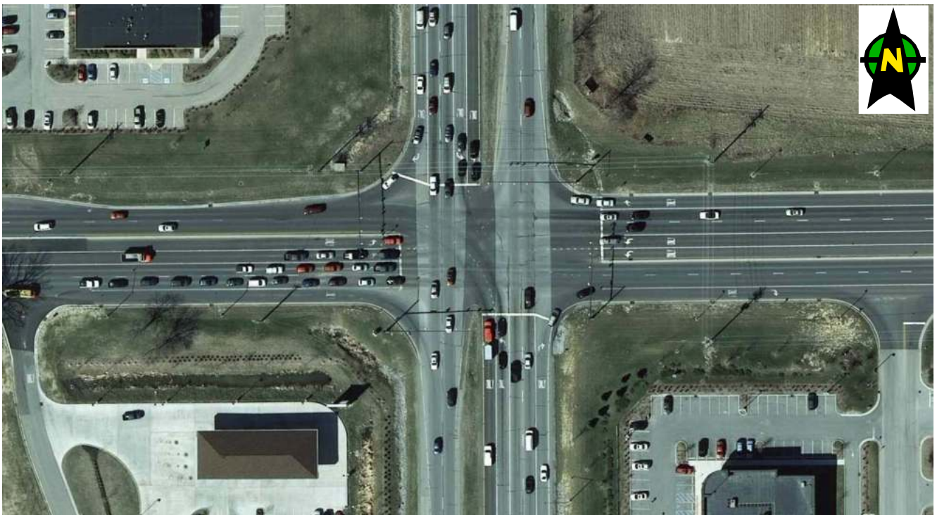
Intersection of SR 37 and 146th Street
