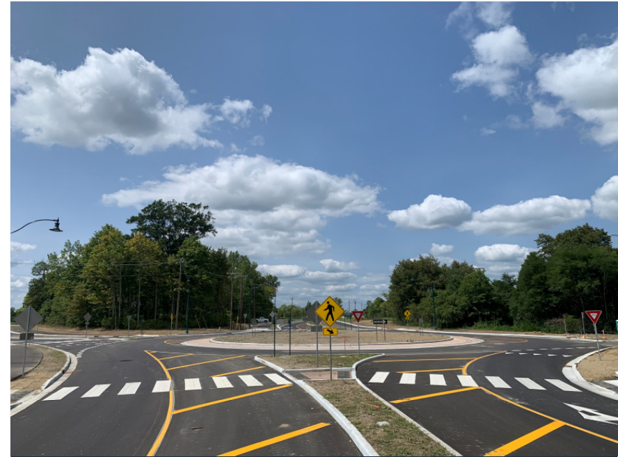
Newly constructed 126 th and Southeastern RAB
