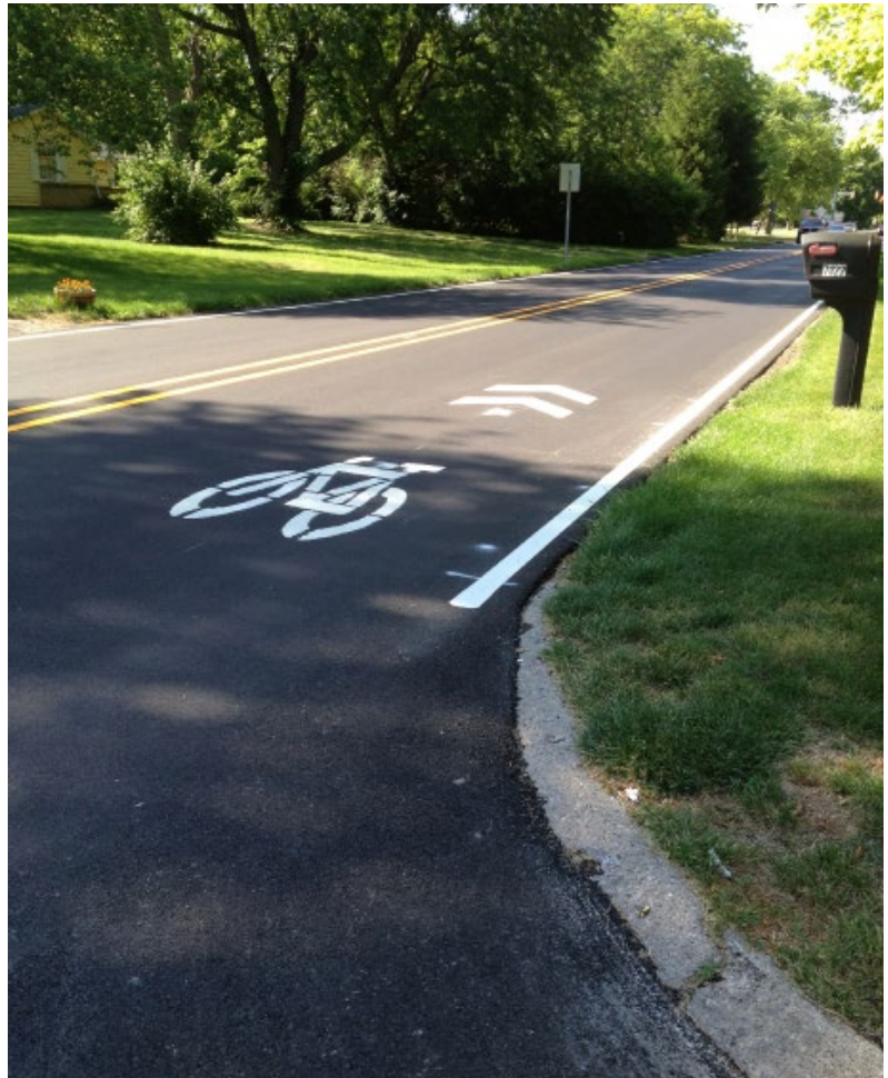
Currently, Fishers does not have any designated shared lanes. This image is of a residential street with bicycle shared lane markings in Indianapolis.
