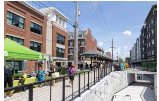
Nickel Plate Trail at 116th Street
