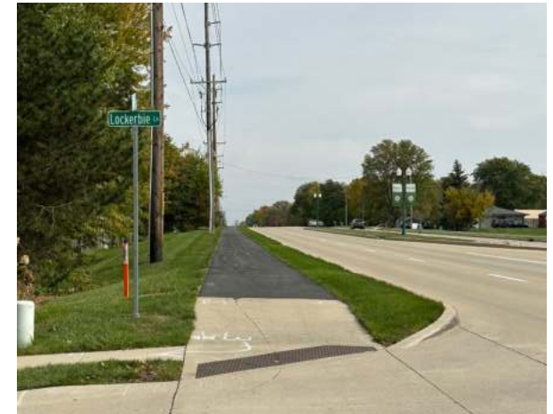
126th Street Existing Conditions
