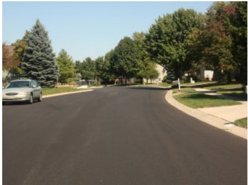
Turkel Drive is an example of a typical local street with curb and gutter, sidewalks on both sides, and room to park on either side of the road.
