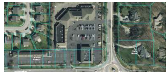
An aerial photo of the commercial buildings at the northwest corner of Fall Creek and Brooks School Road demonstrate how the shops and restaurants offer a nice amenity to neighboring residents while also providing a buffer from the arterial roads.
