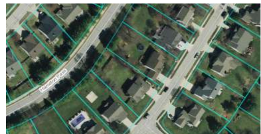
This aerial image of residential lots in Hamilton Proper neighborhood is typical of low density suburban residential lots.
