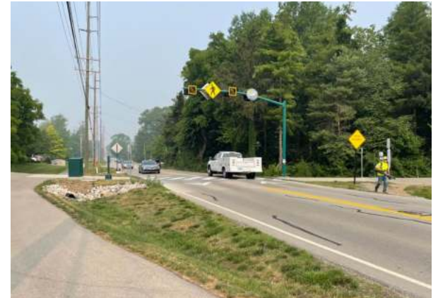
Nickel Plate Trail at 106th Street
