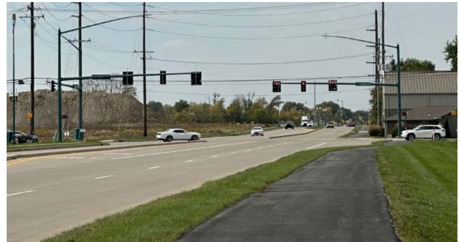
126th Street Existing Conditions
