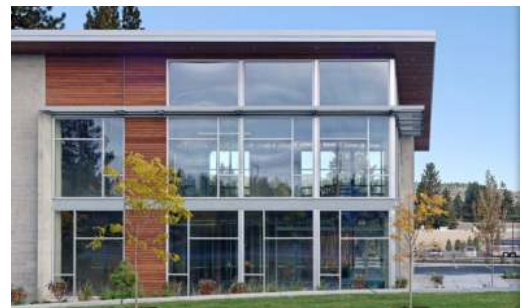
The photo above is an example of the building scale and aesthetic that is envisioned in the Flex Employment category. Buildings are encouraged to use innovative materials and construction methods that allow for adaptation to changing needs.
