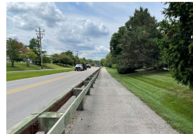
Existing Protected Bike Path on Brooks School Road
