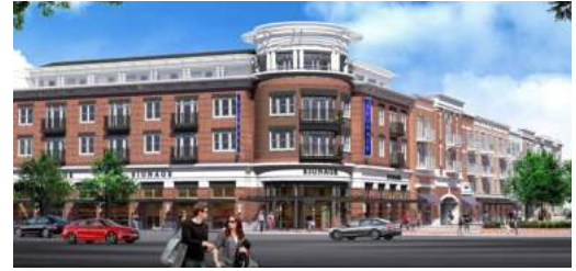
The Depot at Nickel Plate is an example of a regional mixed use district, with retail and residences in the same structure. The garage parking provides opportunity for a building forward design and walkable streetscape.
