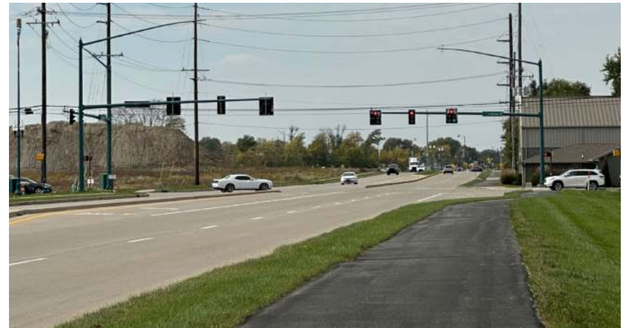
126th Street Existing Conditions
